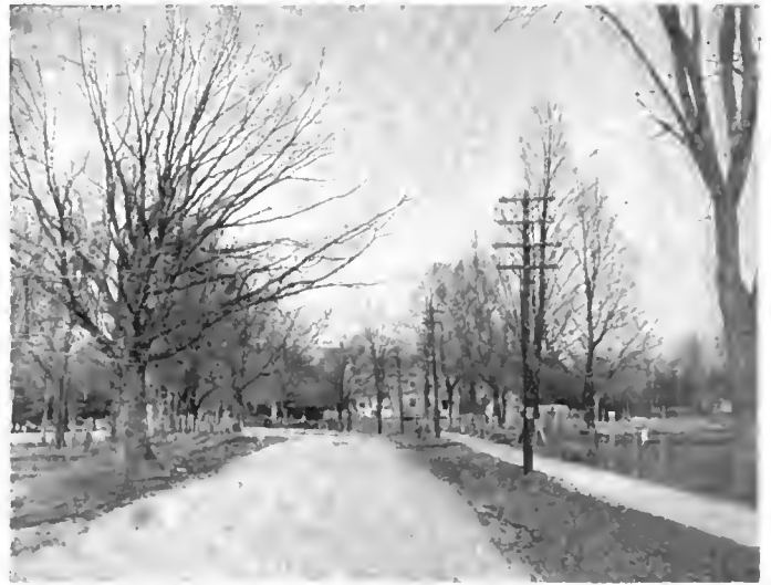
A Modern Road Surface that Has Been Treated with Tarvia
